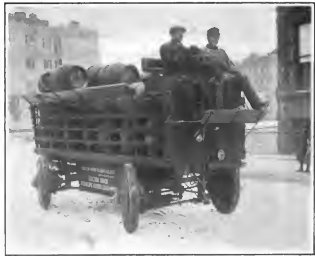
ALL WHEELS SET AT SAME ANGLE FOR OBLIQUE MOVEMENT.
